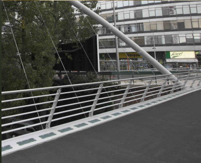
Galvanised metal planks with Hi Grip Plus non slip with Autumn Gold aggregate centred between galvanised open grillage
